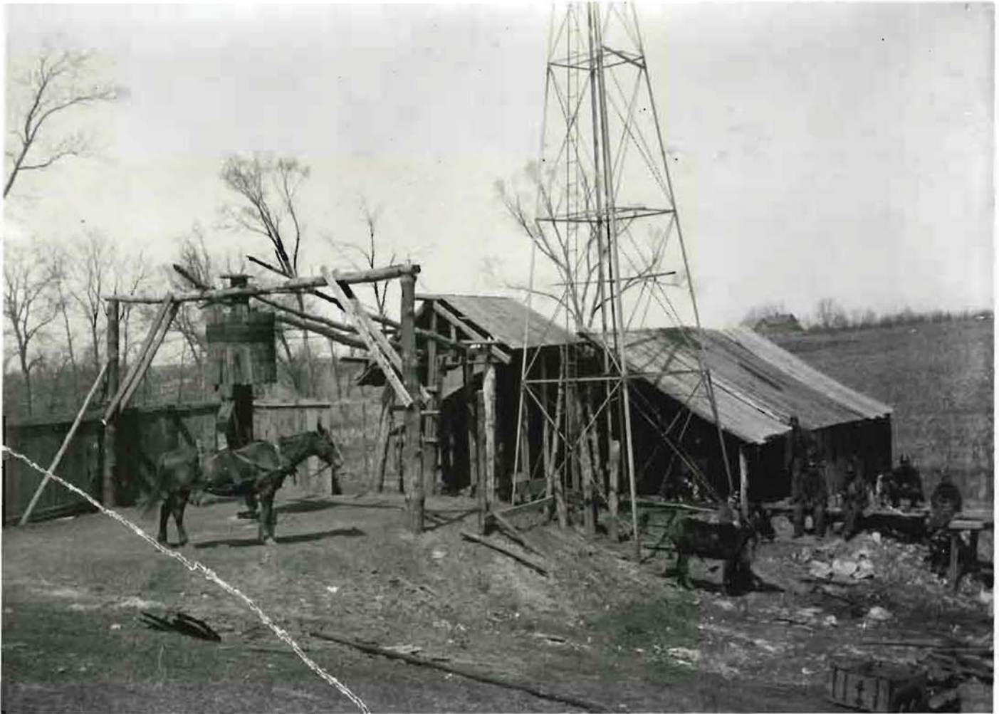
James Brothers Mine at Bevier, Missouri (circa 1911). The horse hoisted coal and supplies up the mine shaft, which is covered by the sheds. The mine car in the right foreground was used underground to haul coal from the working face to the main shaft.
