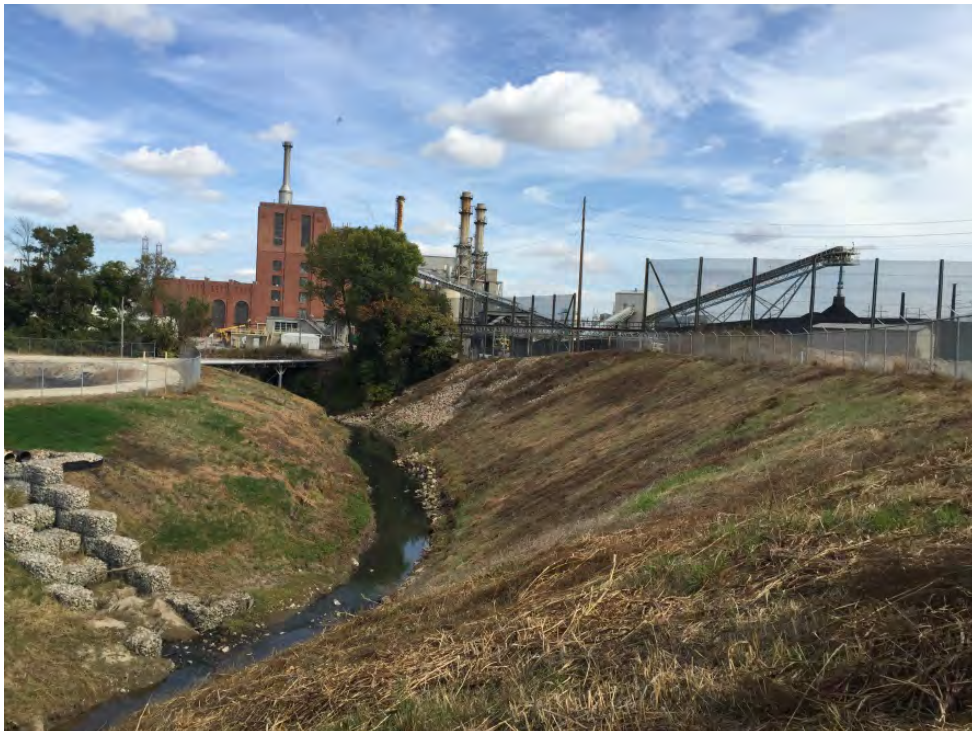
Photograph No. 10 North Berm Downstream Slope
