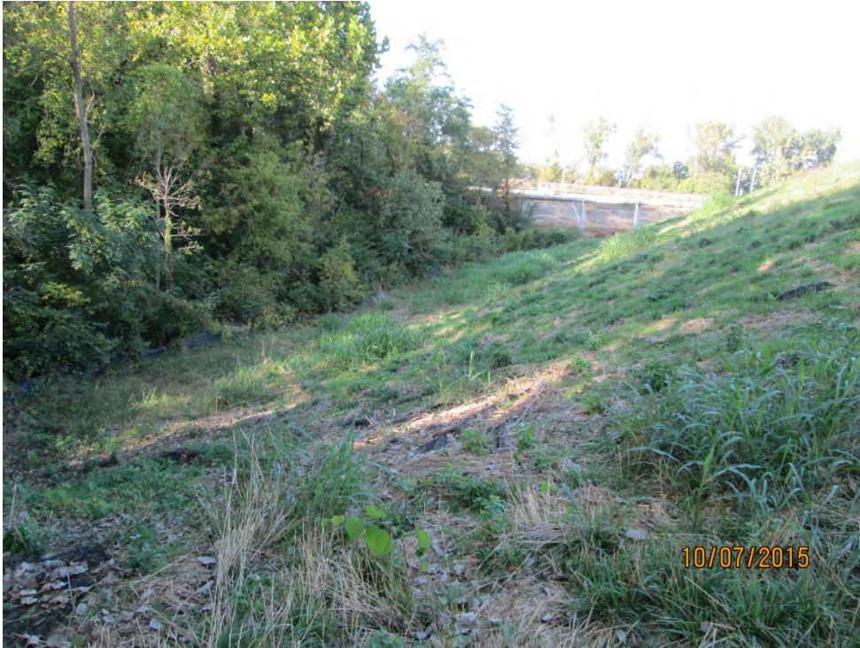
Photo No. 11 West Berm Downstream Slope
