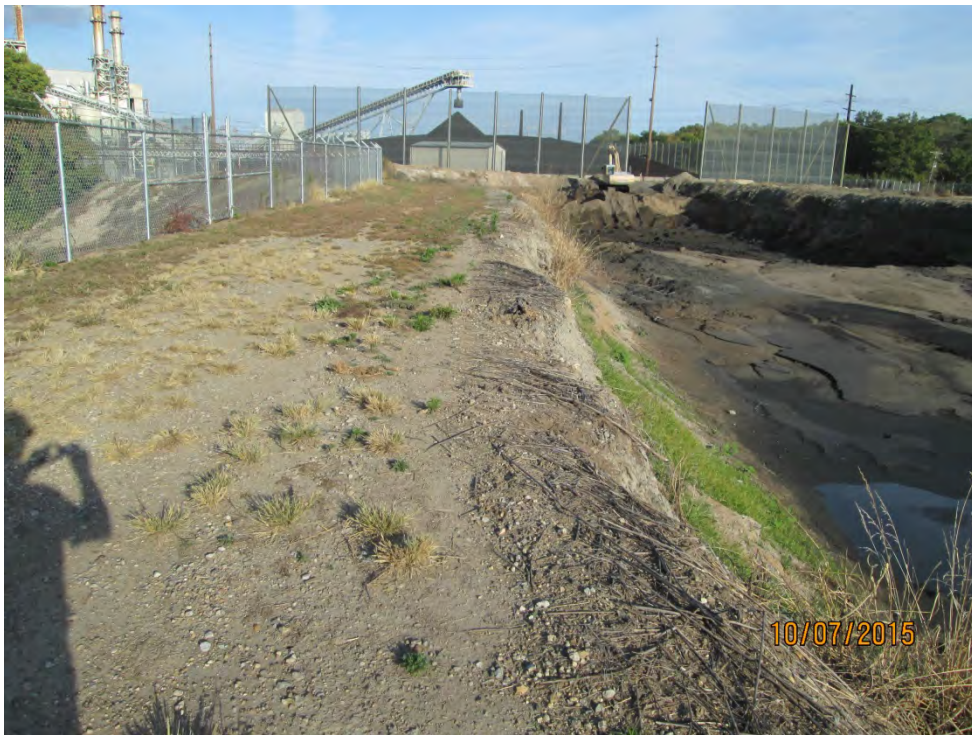
Photo No. 6 North Berm Crest
