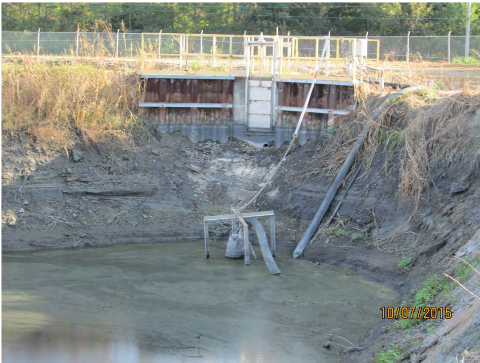
Photo No. 22 Intake Structure
