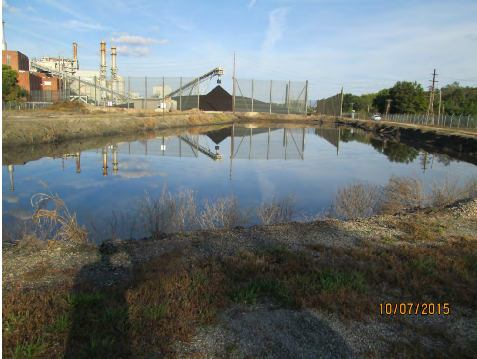
Photo No. 1 South Pond
