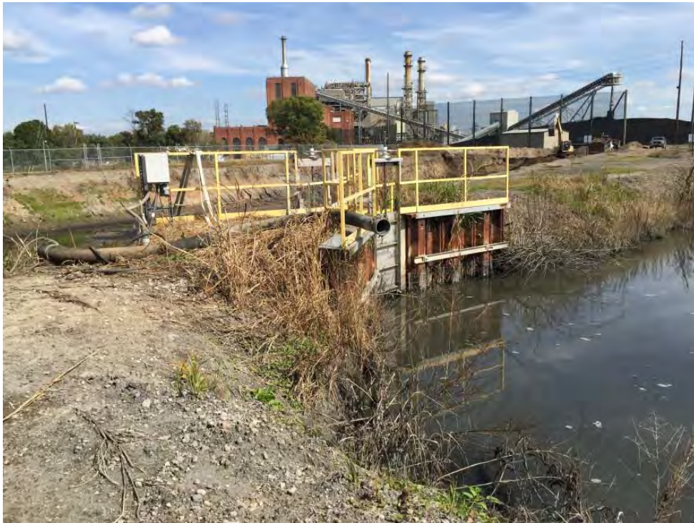
Photo No. 20 Intake Structure
