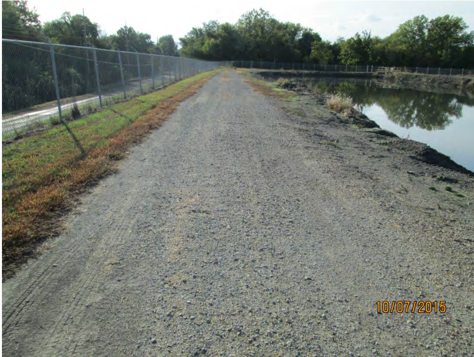
Photo No. 5 South Berm Crest
